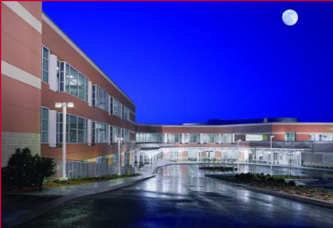
San Mateo County Medical Center
